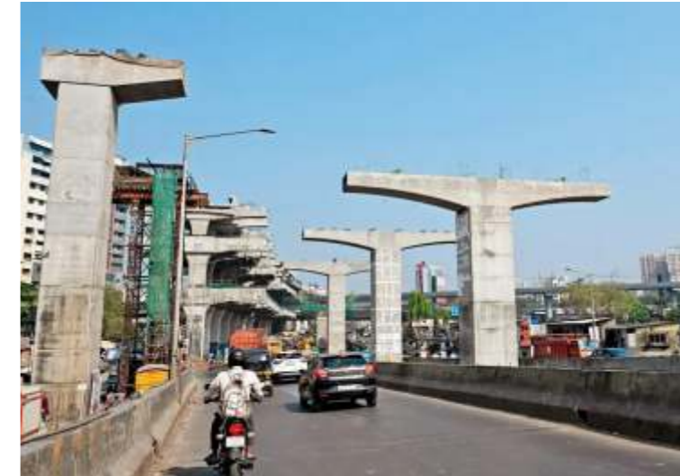
Ongoing road widening, new flyovers, and improved east-west linkages
