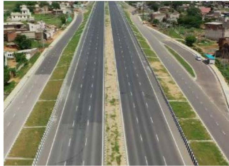
Ongoing Virar-Panvel-Alibaug Multi-Modal Corridor
